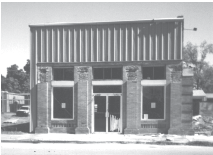
Goshen’s town hall building as it appeared just prior to it being torn down for construction of the new facility.
